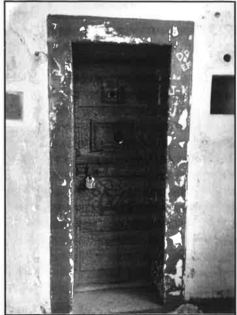
The Cell Door in the West Wing of Kilmainham Convict Depot
