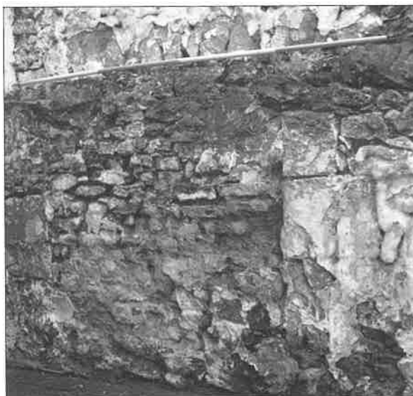
Plate 2: detail of blocked possible window embrasure at ground floor level.
