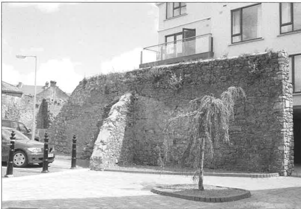
Plate 1: External view of the extant wall at the Dominican Friary site with an early support. (May 2005)
