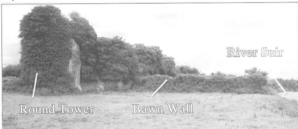
Plate 5. View looking north at the Newcastle castle complex.
