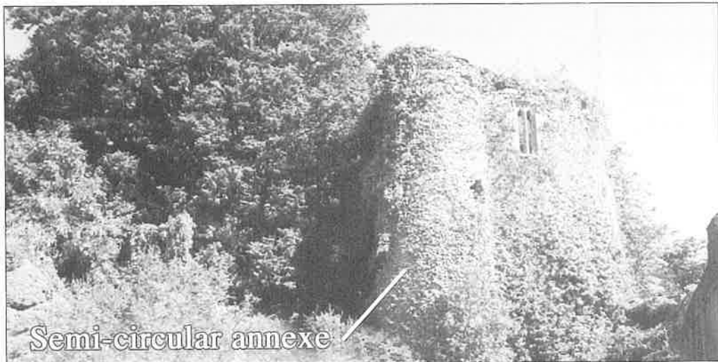
Plate 4. View northeast of the thirteenth century keep and annexe at Ardfinnan.
